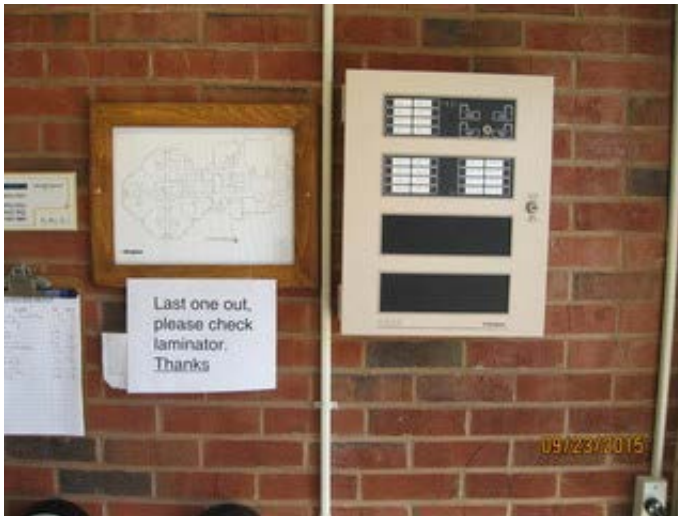
Fire Alarm Remote Annunciator
