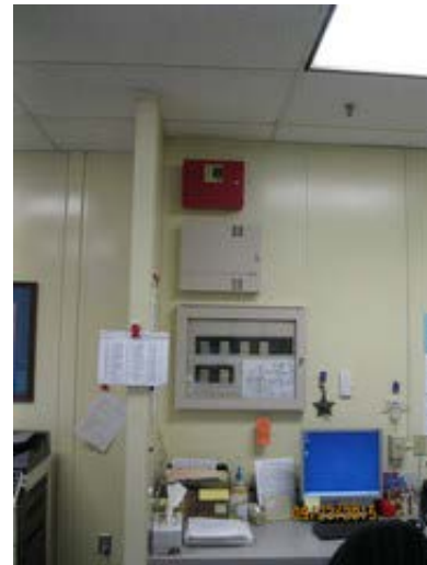
Fire Alarm Control Panel
