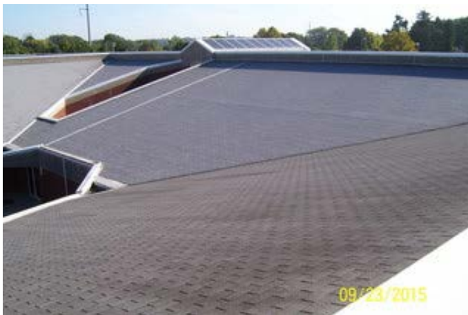
Typical Asphalt Shingles
