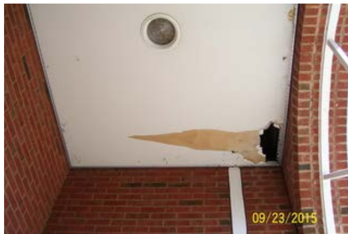
Soffit to be Repaired
