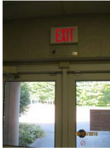
Exit Sign and Door Security Contacts
