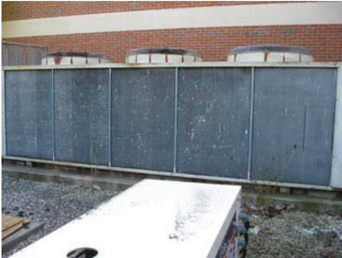
Air Cooled Condenser
