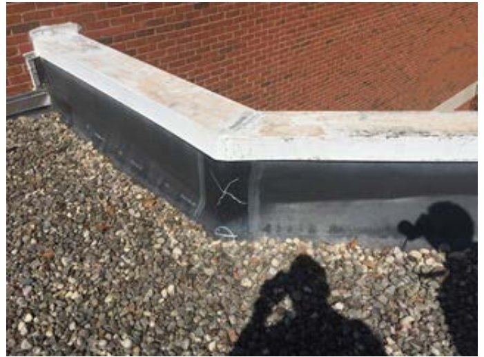
EPDM Roofing and Metal Coping
