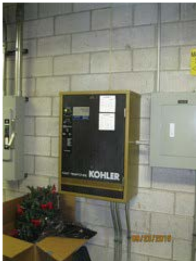
Emergency Panel and Automatic Transfer Switch
