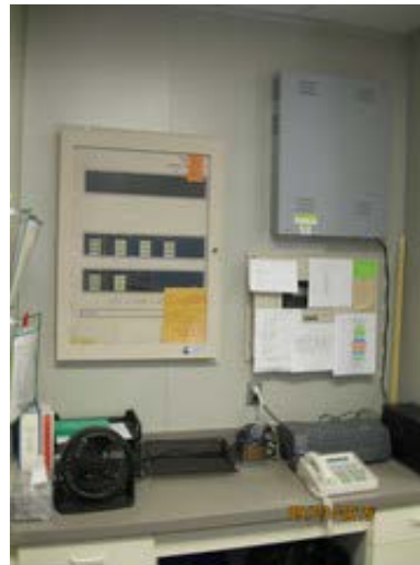
Fire Alarm Control Panel
