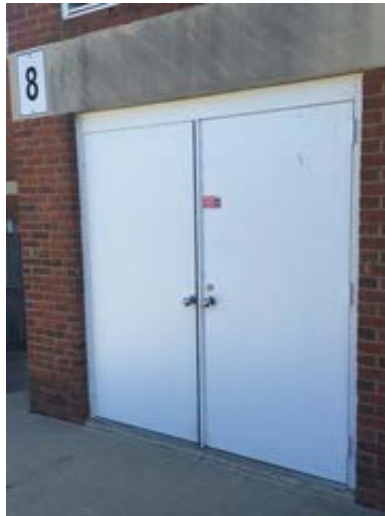
Typical Exterior Door with Inappropriate Hardware
