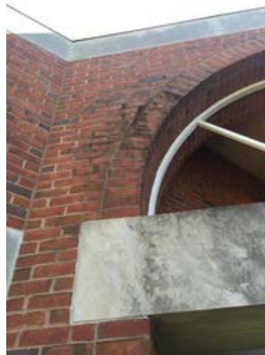
Mold on Exterior Brick and Stone
