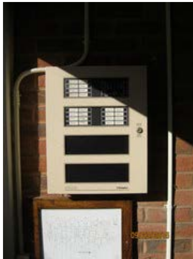
Fire Alarm Remote Annunciator
