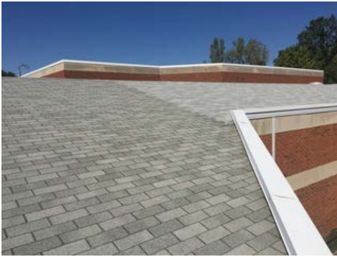
Fiberglass Shingled Roofing
