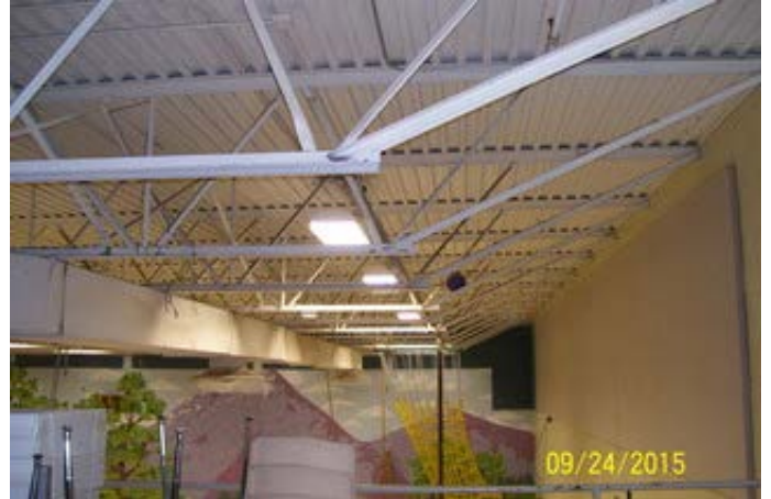
Typical Roof Structure
