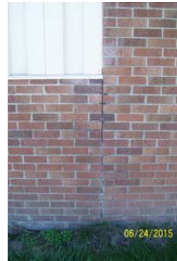
Typical Joint to be Caulked
