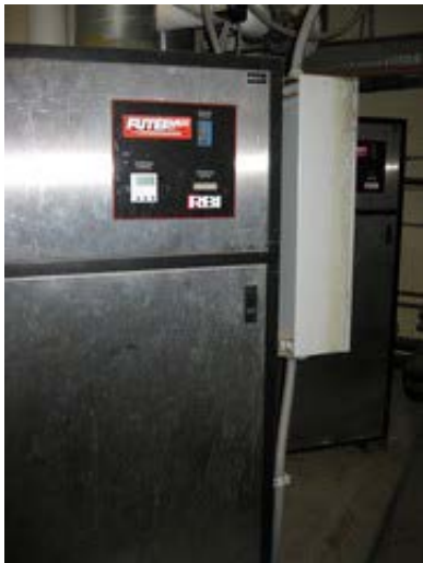
Gas Fired Boiler
