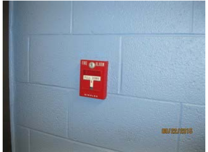
Fire Alarm Pull Station
