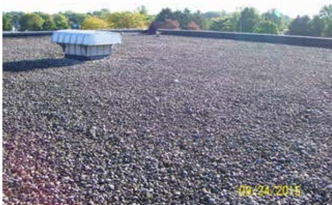
Ballasted Roof at Gymnasium
