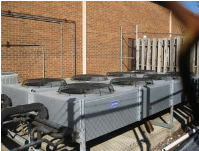
Air Cooled Condenser
