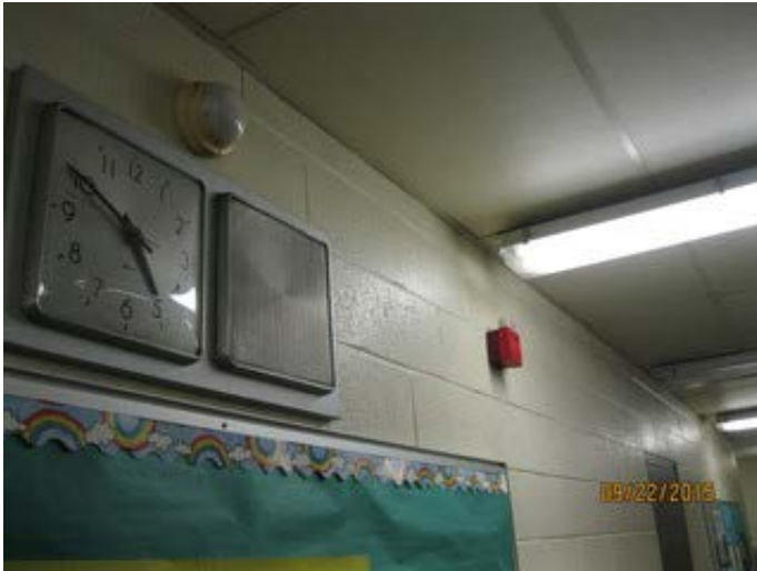
Fire Alarm Horn Strobe
