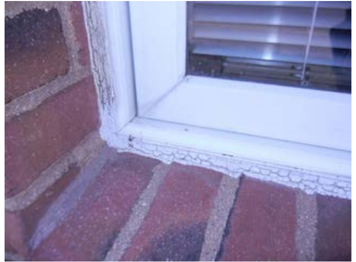
Poor window seal condition
