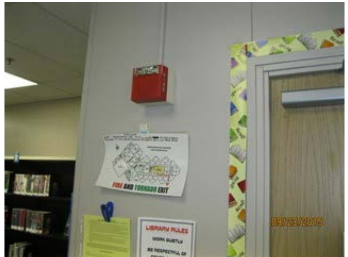
Fire Alarm Horn/Strobe
