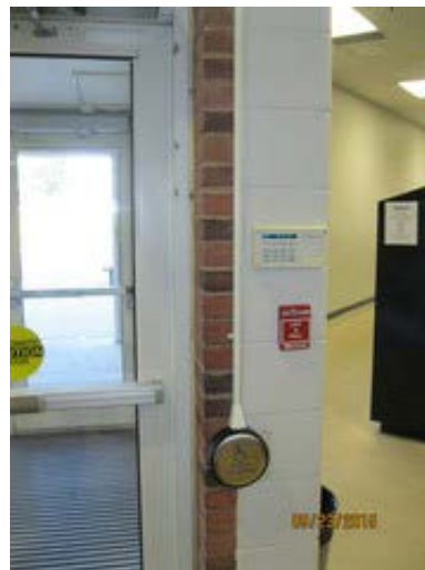
Security System Keypad and Fire Alarm Pull Station
