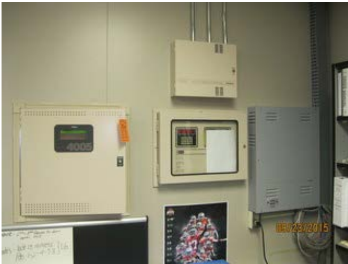
Fire Alarm Control Panel and Central Time Panel
