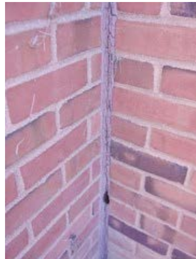
Exterior caulking in poor condition
