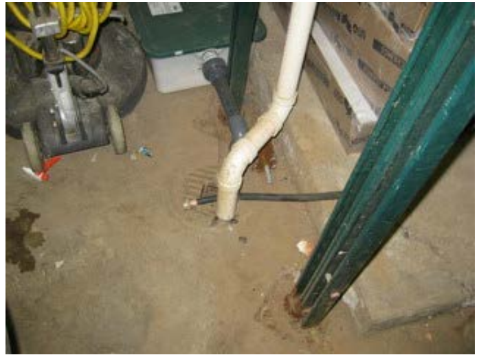
Exposed Waste in Boiler Room
