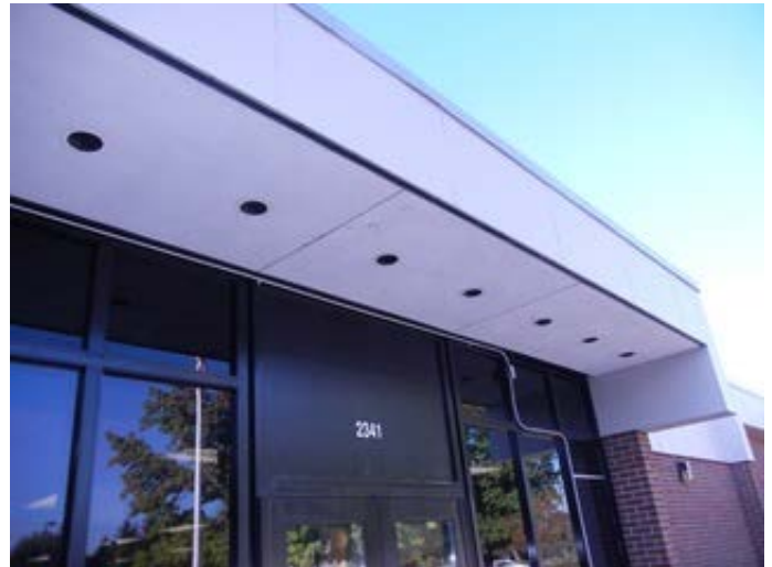
Soffit and Fascia Panels at Main Entry
