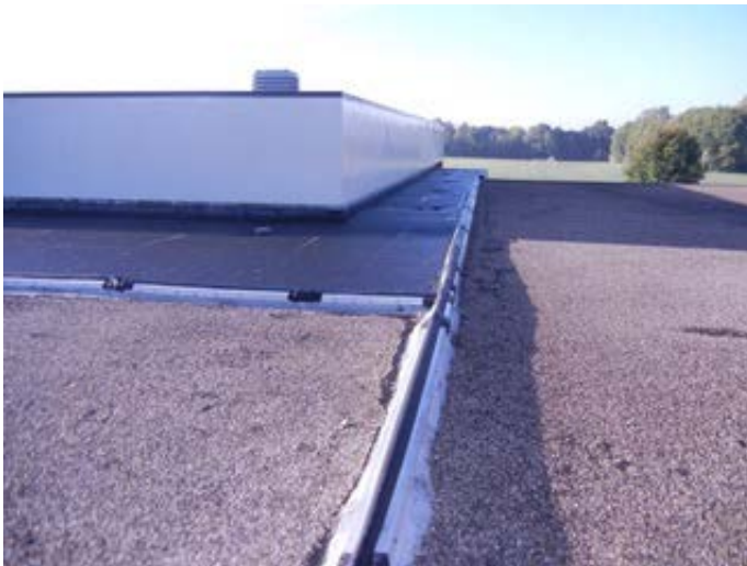
Built Up Roof in Foreground and EPDM Roof in Background
