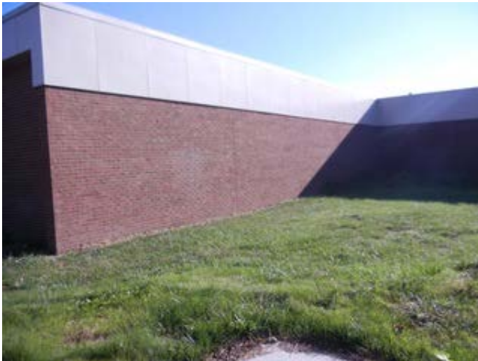
Brick Exterior Wall with Fascia Panels
