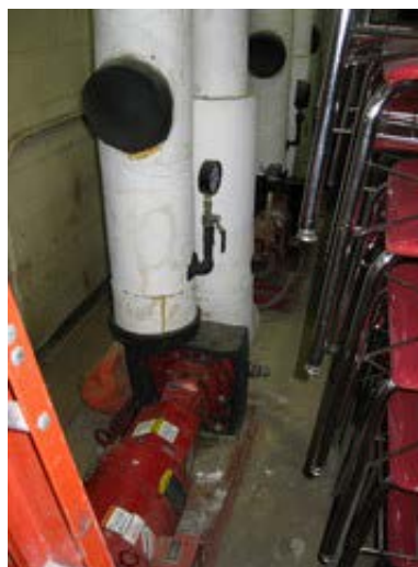
Heating Hot Water Pumps
