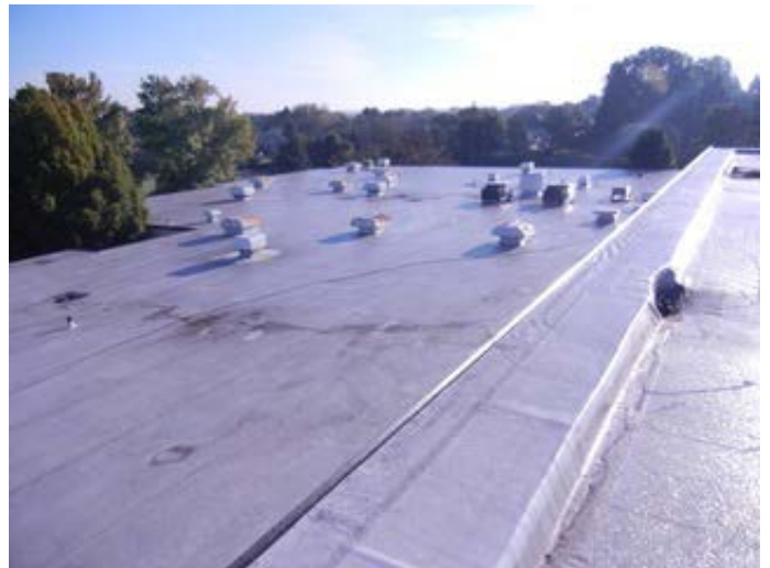
Thermoplastic Roof System
