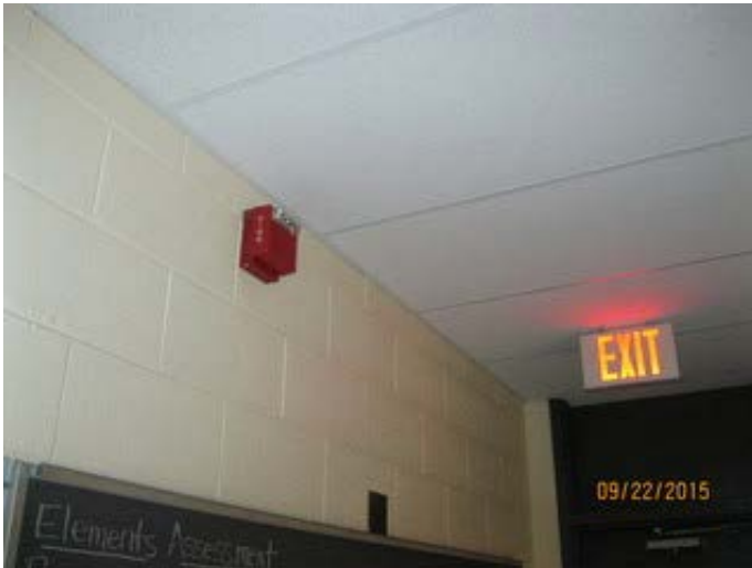
Fire Alarm Horn Strobe
