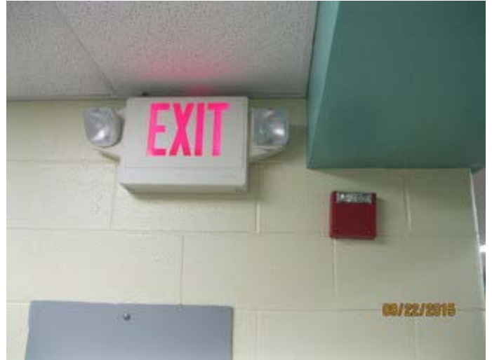
Combo. Exit Sign/Remote Heads/FA Horn Strobe
