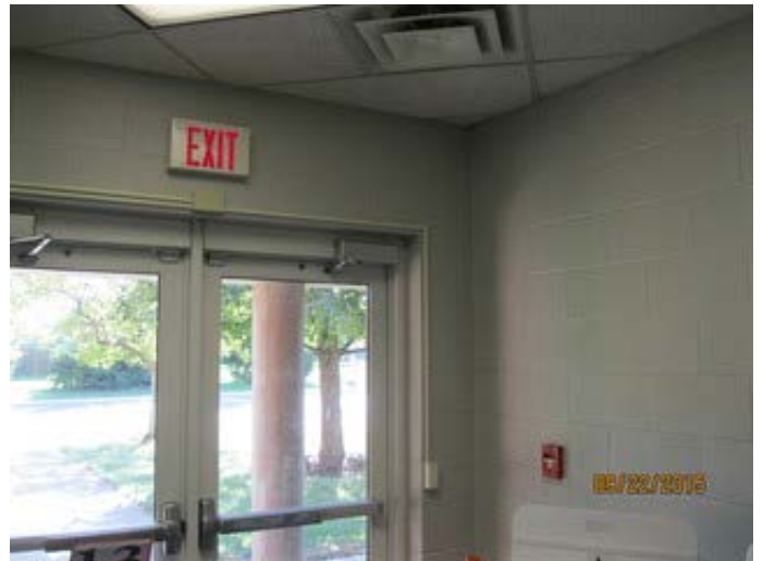
Corridor Exit Sign/FA Pull Station/Security Door Contacts
