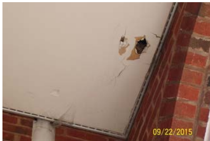
Typical Soffit to be Repaired
