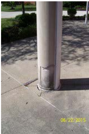
Typical Column Cover to be Replaced
