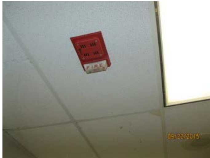
Ceiling Mounted FA Horn Strobe
