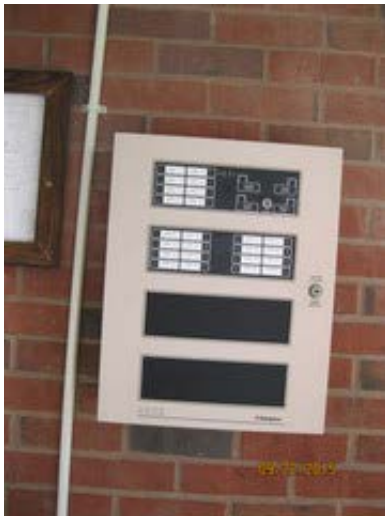
Fire Alarm Remote Annunciator
