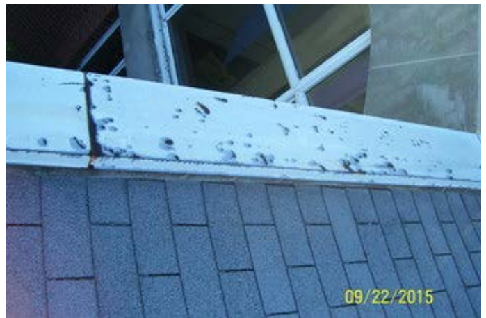
Typical Coping to be Replaced
