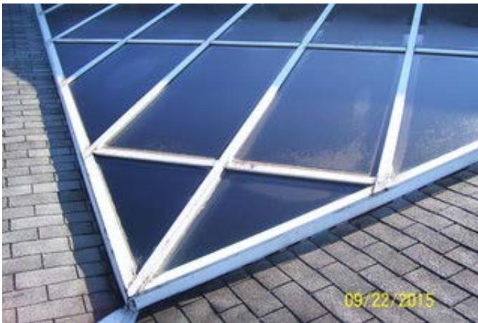
Typical Skylight System to be Replaced
