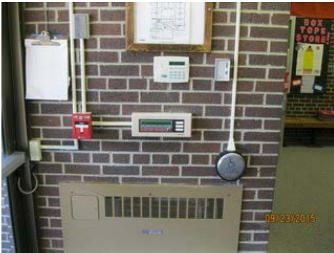
FA Remote Annunciator/Security System Panel
