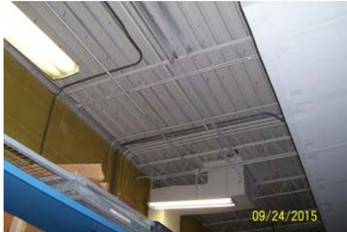
Typical Deck and Joists
