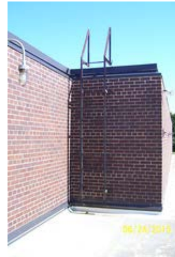
Access Ladder to be Replaced
