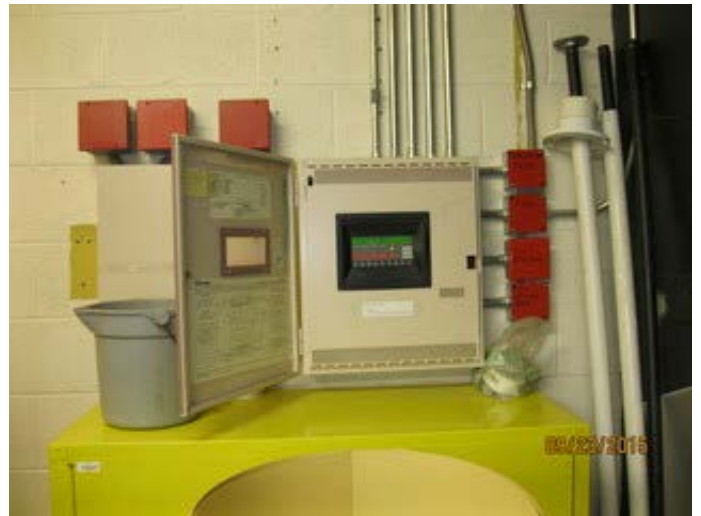
Fire Alarm Control Panel
