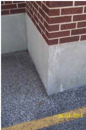
Minor Cracking to be Repaired
