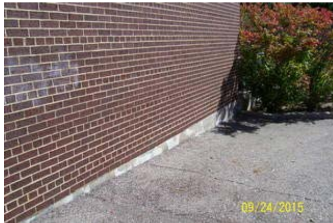
Minor Spalling to be Repaired
