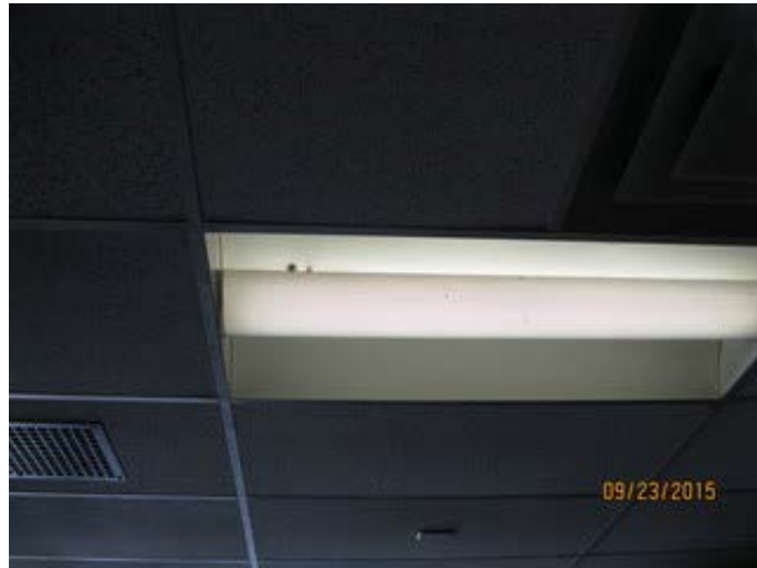
Recessed Lighting With Battery Pack
